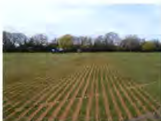
Sand grooves installed at 260 mm centres
