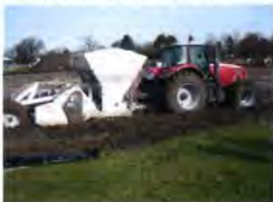
Installation of ground stabilisation treatment
