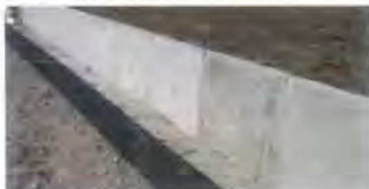
Pre-formed ditch channel simplifies construction
