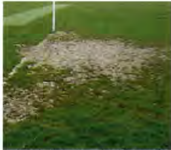
Poorly constructed and / or maintained playing surfaces are dangerous, affect quality of play and limit use
