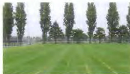
Combined pipe and slit drainage will significantly improve the drainage of most pitches
