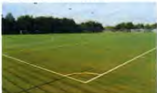
Sand-filled pitch with 23 mm pile onto a 15 mm shock pad for hockey and for football training
