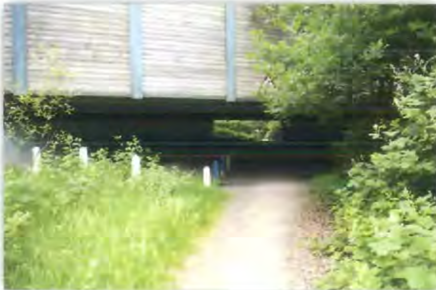
Photograph 4-2 M25 underpass looking south
