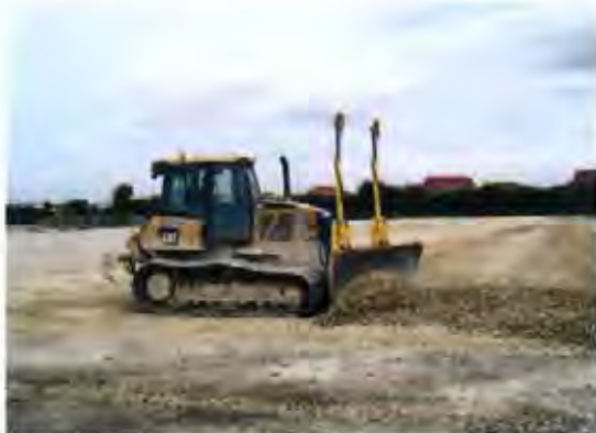
Laser-guided grading of a pitch
