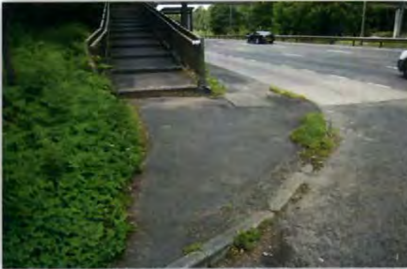
Photograph 3-3 Existing footway and access to footbridge at Elm Lane
