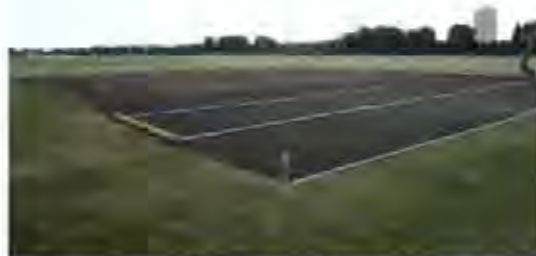
Precise placement and consolidation of cricket loam is crucial to the success of cricket square construction
