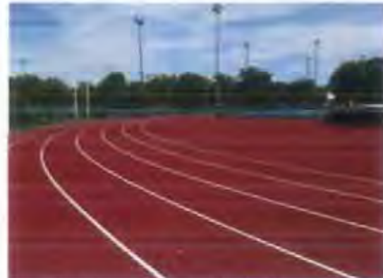
Resurfaced porous macadam track
