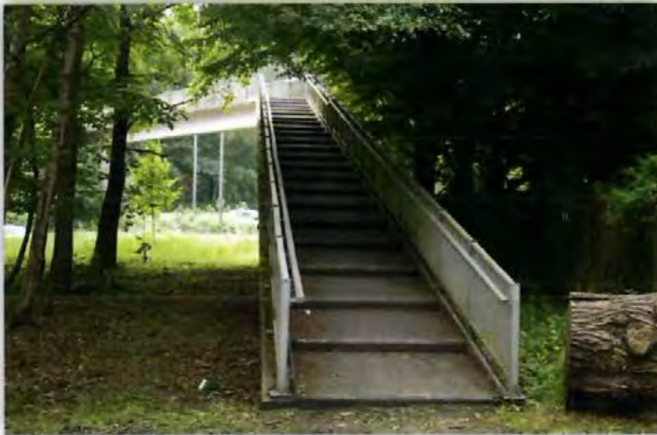
Photograph 3-4 End of Footbridge on the Wisley Side of A3
