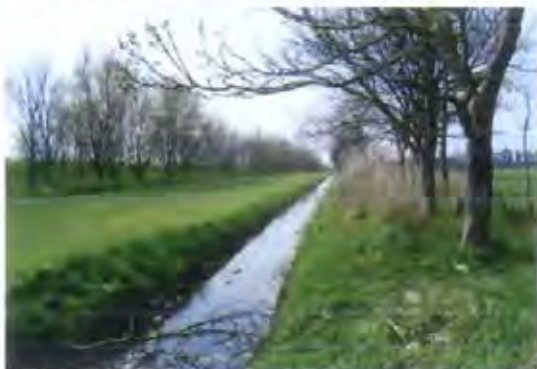
Adjacent water course can provide a convenient means of achieving efficient drainage provided that a 'land drainage consent' can be obtained
