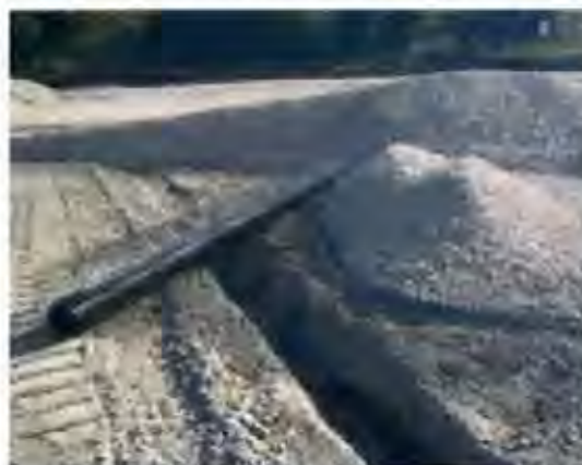
Plastic mesh within stone layer
