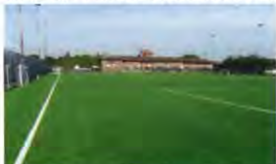
Resurfaced pitch with 60 mm 3G long pile onto a 15 mm shock pad for football and for rugby training
