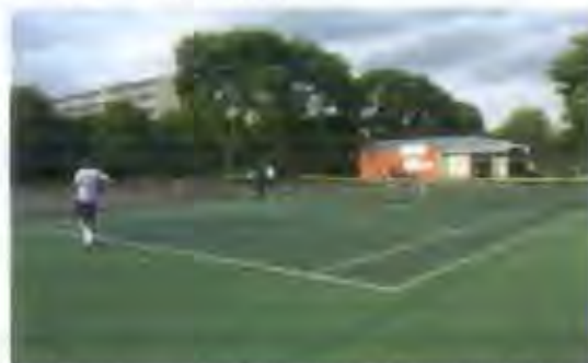
Acrylic tennis court surfaces painted on a macadam base
