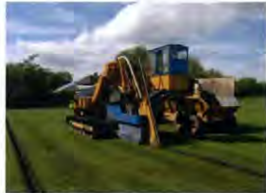
Installing pipe drainage in a new pitch
