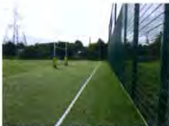
A 3G rugby pitch with carpet extending right up to the fence
